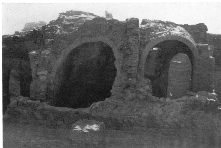
4. Vaulting of III-O and N; looking east
