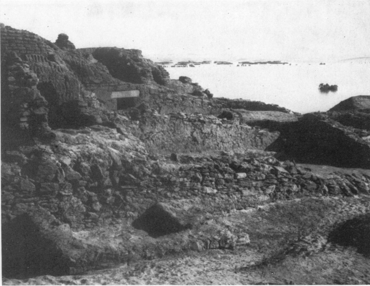
1. Room I-I with I-BB in foreground; looking east
