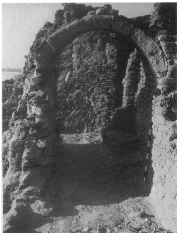
3. Room II-MM, showing possible entrance to II-P at rear
