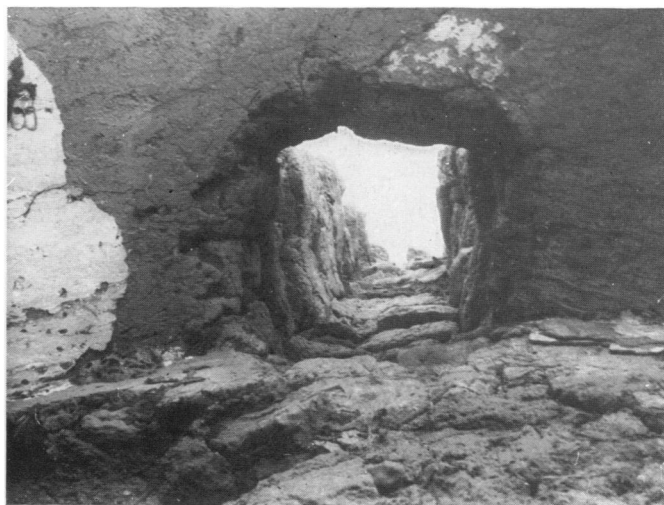
4. Communications shaft in soffit of archway in south wall of II-B (see 2. above)
